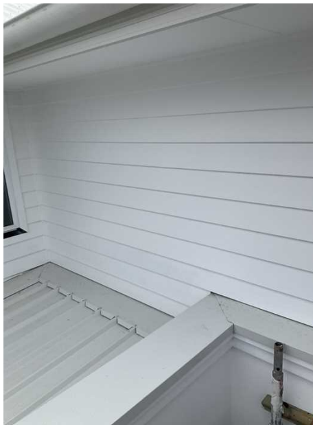
+ Example of cladding
