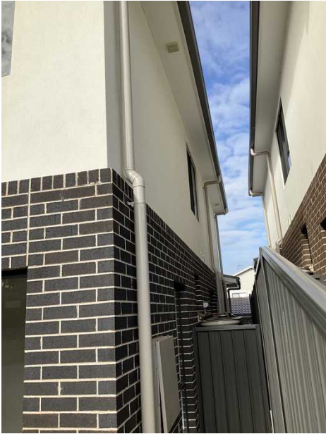
Showing example of Brickwork completed
