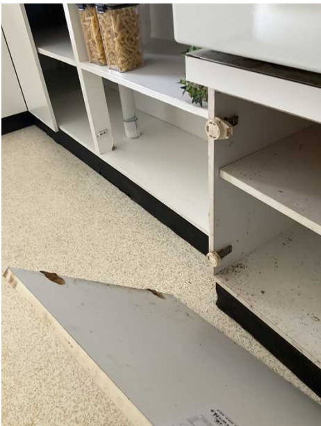
+ Example of kitchen door falling off when I opened it. Timbers are old and deteriorated. Complete new kitchen required in the very near future.
