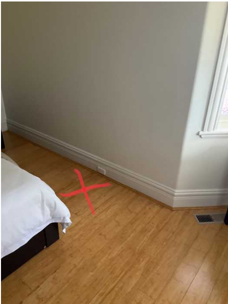
+ Flooring or floor joist has no support to underside. Floor movement very evident. Likely cause by sagging or leaning piers. Entire house has undulated flooring. Engage engineer and seek advice to prevent further deterioration.
