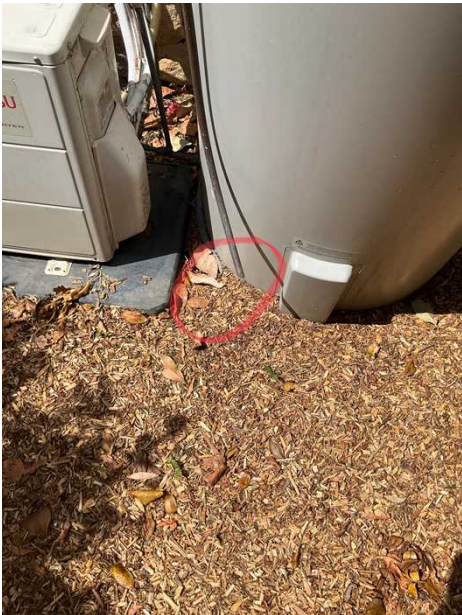
Example of hot water overflow.
