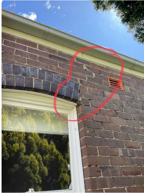
+ Example of large crack above window of bedroom 2
