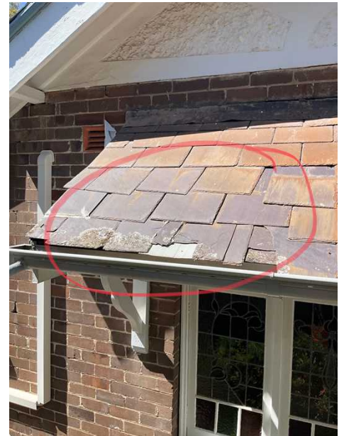
+ Example of broken and missing slate tiles. Some tiles have been siliconed together,
