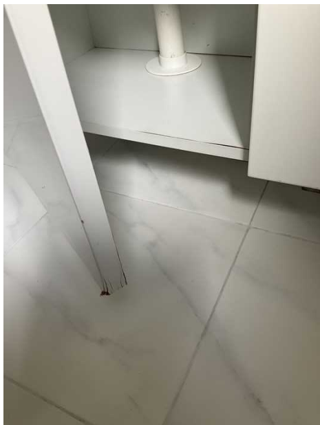
Water damage to vanity, recommend carpenter to repair/replace to prevent further deterioration., + Moisture damage to bathroom/laundry vanity.
