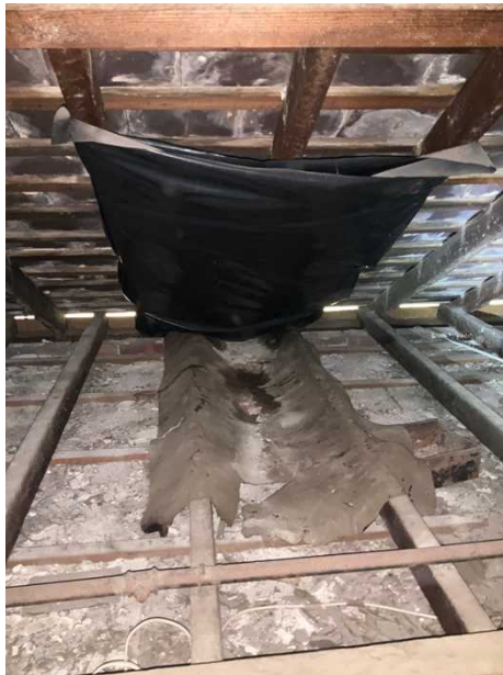
+ Plastic installed to what seems to be a way to control water ingress. Engage roofer for water testing to identify leaks and do suitable repaired to prevent water ingress.
