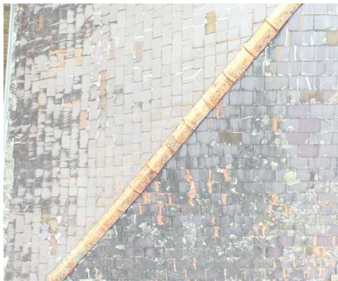
+ Example of drone images. Roof looks aged and weathered. Engage roofer for repairs and maintenance.
