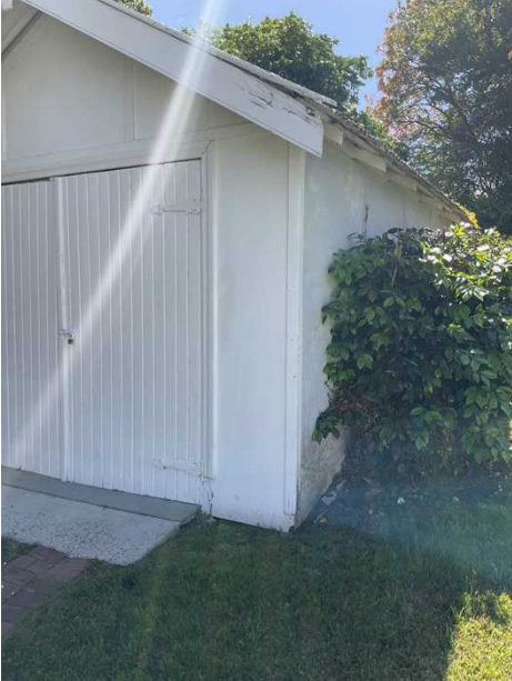
+ Walks to garage are likely asbestos based. Ensure testing of lining is completed prior to any work or removal of sheets. Asbestos is life threatening and all care should be taken when working with this material.
