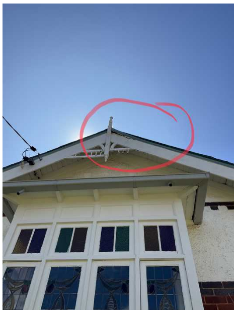
Aged and deteriorated fascia- Engage a carpenter to repair/replace to prevent further deterioration and damage.
