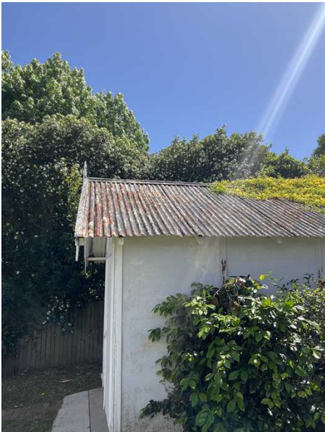
Rust to parts of the roof. Recommend engaging a roofer for repairs to prevent further deterioration and damage., + Rear garage location.
