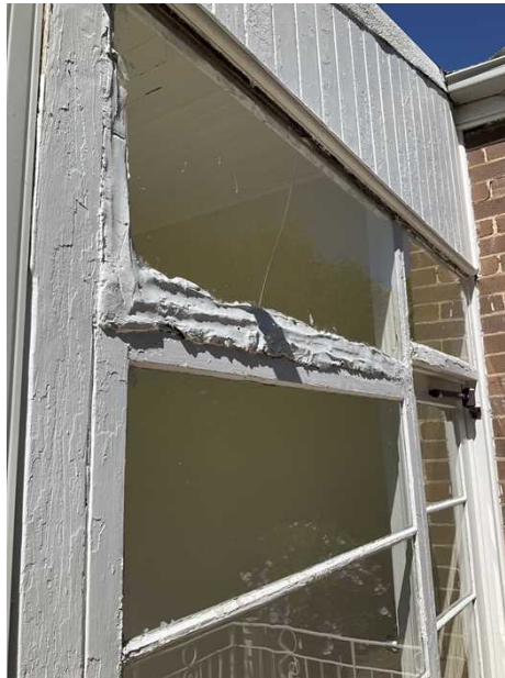
Weathered timbers to parts of the windows. Recommend a carpenter for repairs to prevent further deterioration., Cracked and missing putty to parts of the windows. Recommend a glazier to repair/replace to prevent further damage., + Sunroom location.
