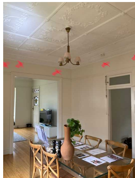
+ Example of cracking to dining room. Cracks recently repaired but will return in the near future.
