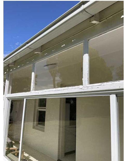
+ Example of weathered window frames to sunroom.
