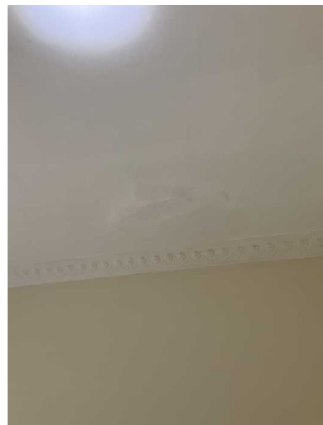
+ Major cracks and ceiling sagging to ceiling in kitchen. As per other rooms. Ceiling is 120 years old and reached its life span. Home has major foundation movement. Will require ongoing maintenance to control cracking.
