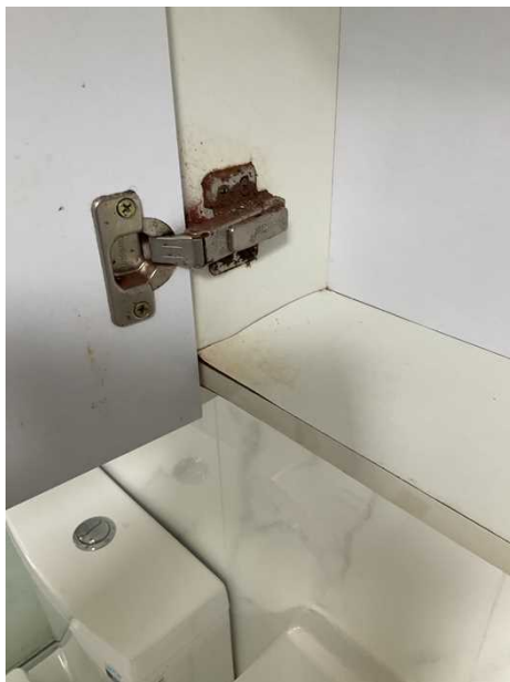
+ Moisture damage to shaving cabinet in bathroom/laundry.
