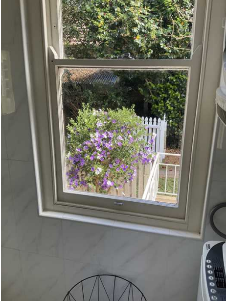
+ Example of some windows that do not open likely due to been glued with paint.
