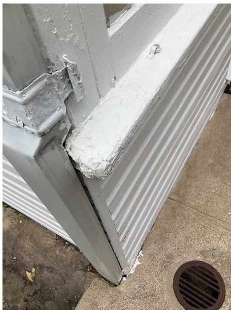
Example of wood rot to window frames.
