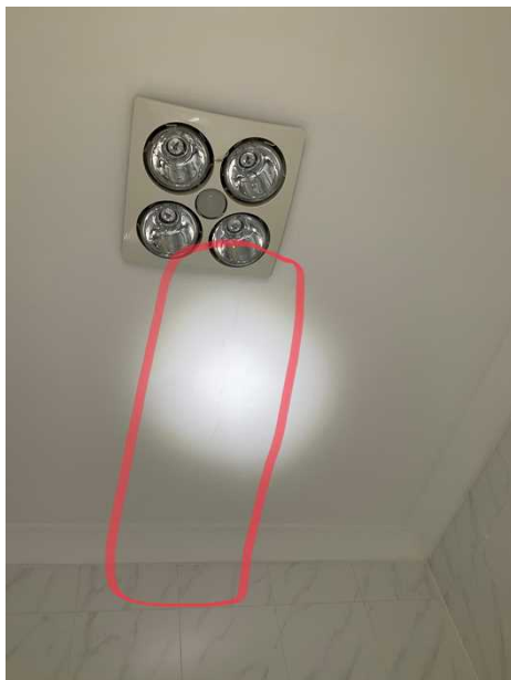
+ Ceiling in laundry bathroom has been replaced in the past. Evidence of large crack which has been repaired. This aligns with the movement of the foundations causing cracks throughout ceilings, walls and undulated flooring.
