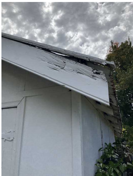
Example of wood rot to fascia boards.
