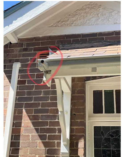
Example of no down pipes connected. Moisture is conducive to termites. It's important to prevent excess moisture around the property not to attract termites.
