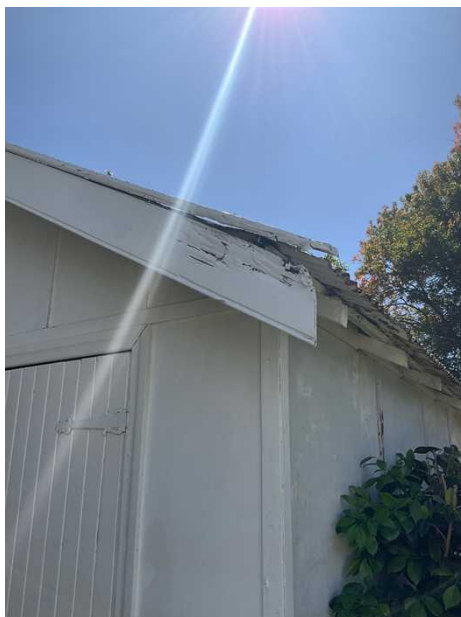
Aged and deteriorated fascia- Engage a carpenter to repair/replace to prevent further deterioration and damage., + Located at rear garage.
