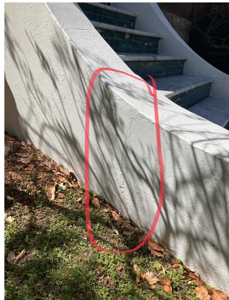
+ Cracking to porch stairs. Engage engineer for advice to prevent and control further cracking.
