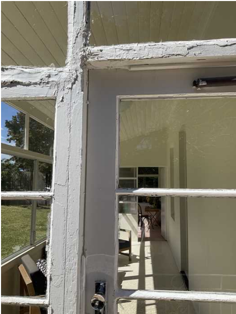
+ Rear sunroom door is weathered and deteriorated as is the door jamb. Extensive work required throughout to make good of sunroom.
