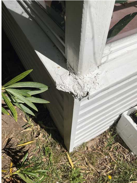
+ Example of more wood decay to sunroom walls. Engage carpenter for repairs to prevent further deterioration.
