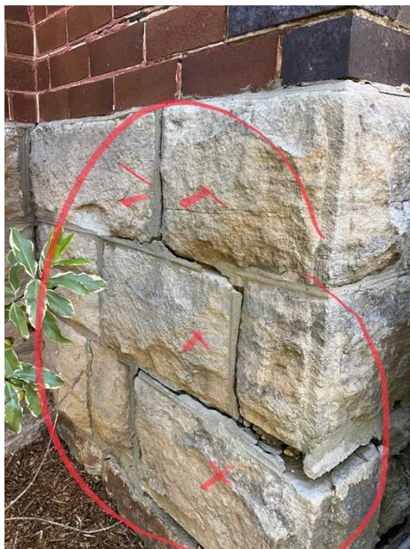
+ Cracking to sandstone foundation walks. Engage engineer for advice to repair and prevent further deterioration.
