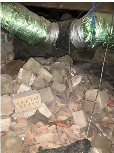
+ Example of blocked access to entire subfloor by ac ductwork
