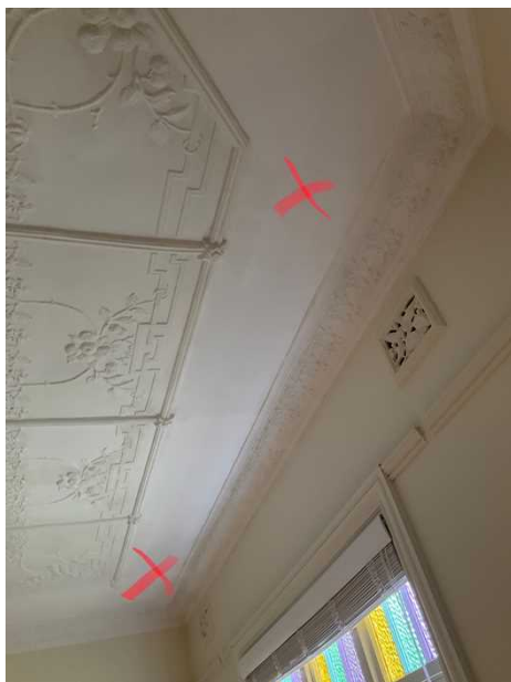
+ Example of repaired movement cracks to ceiling. Located in dining area.
