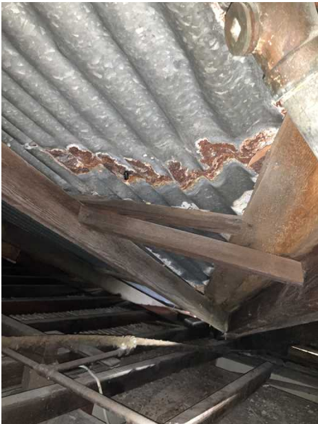
+ Rusted corrugated sheets above kitchen , bedroom 2 and Laundry. Undetermined if any water ingress during rain. Engage roofer for water testing. Likely to require replacement in the near future.
