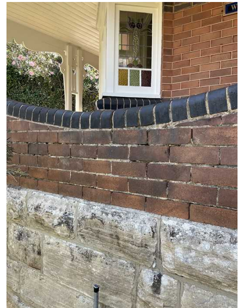
+ Cracking and mortar breakdown to front porch brickwork. Engage bricklayer for repointing to prevent further deterioration.
