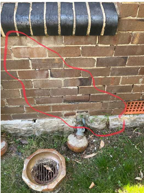
+ Cracking to outside window of bedroom 2. Engage engineer for advice to prevent further deterioration.
