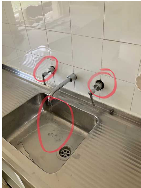
+ Unsealed Tap hardware within wall. Engage joint sealer to seal gaps to prevent water ingress within walls. Engage plumber to replace seals in taps to stop leaking taps.
