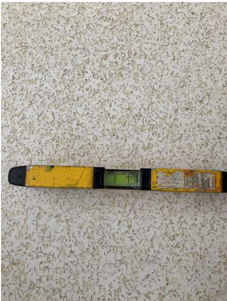
+ Flooring to sunroom and study has major fall. Engage builder or engineer for advice.
