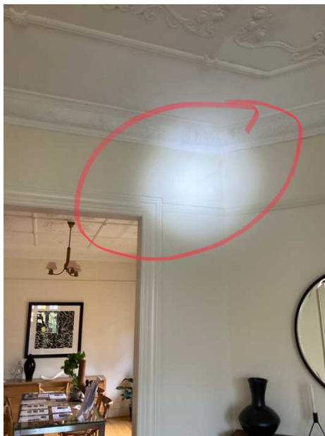
+ Example of cracking to living room above fireplace.
