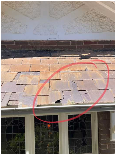
+ Slate tiles have slid down and not providing protection in areas of the roof. Engage specialised roofer for repairs to prevent water ingress.
