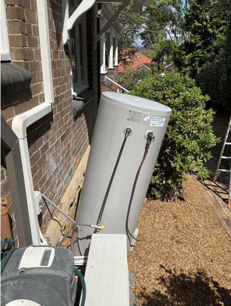
+ Subsiding water heater. Engage plumber to remove and install suitable base for water heater to prevent subsidence and leaning.
