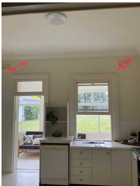
+ Example of cracks to kitchen. As per most cracks in the house they have tried to cover up. These are major cracks and will return in the near future.
