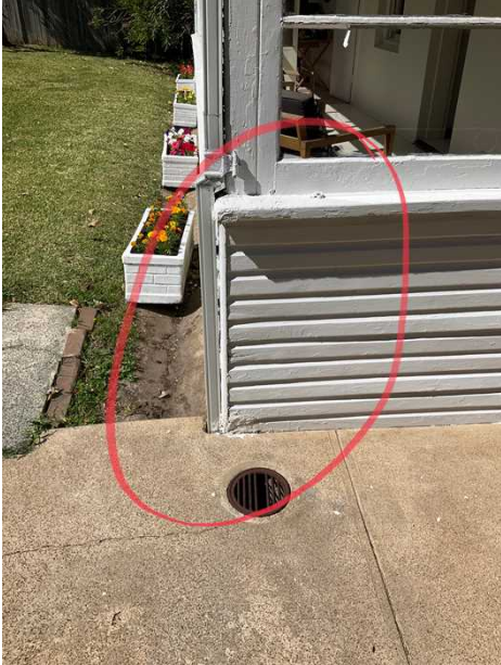
Weathered timbers to areas. Recommend a carpenter to repair or replace as required to prevent further deterioration., + Has been poorly patched by the painter.
