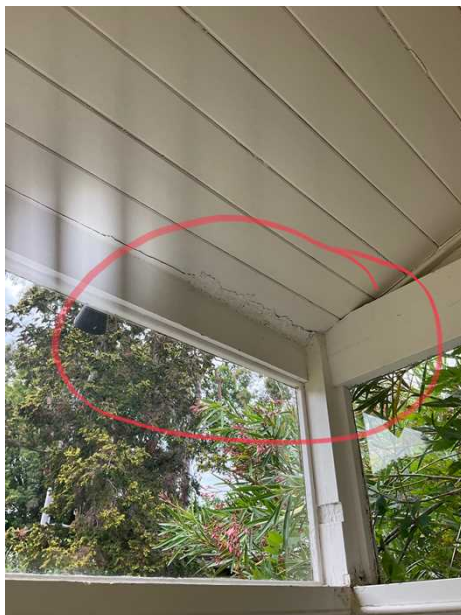
+ Example of poorly repaired timber ceiling in study.
