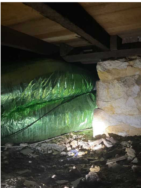
+ No access due to AC ducting blocking access hole. On partial inspection under living room. Property & Timber Pest Report.
