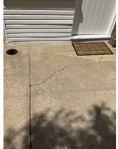
Cracked and uneven concrete. Engage concreter for repair/replacing to prevent further deterioration.
