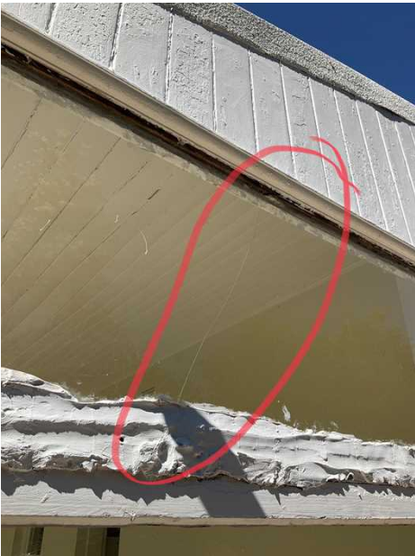
Broken window, recommend a glazier to replace the broken pane to prevent risk of personal injury and water penetration., + Sunroom location.
