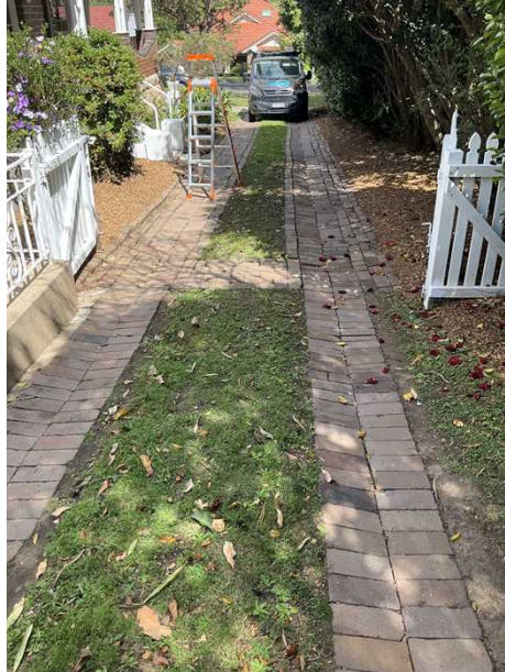
Poor surface drainage-recommend engaging a plumber to rectify ground water issues which can lead to foundation movement., Unevenness of the pavers. Recommend a landscaper for repairs as required to prevent personal injury to footing.
