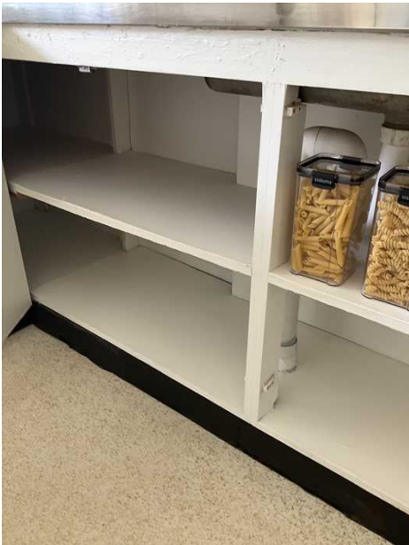
+ Cabinets to kitchen are old and moisture damaged. they have been given a coat of paint to hide deterioration. Missing doors. Will require replacement in the near future.
