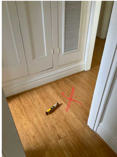
Undulating/uneven floors- recommend engaging a builder for rectification to prevent further deterioration., + Located at corridor of bathroom and bedroom 3.
