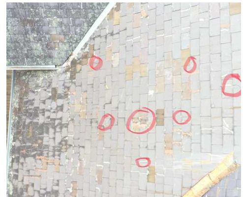
+ Example of cracked or chipped slate roofing. Some tiles have slide. Engage roofer for full inspection and maintenance to prev water ingress.
