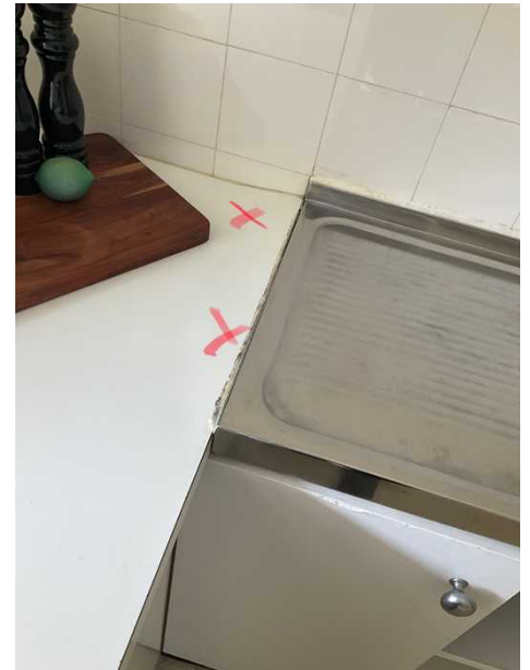
+ Water damaged top to kitchen. Swelling visible. Engage carpenter for replacement to prevent further deterioration.
