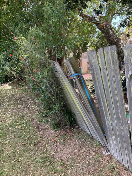
Leaning fence to areas-recommend engaging a fencer to repair and prevent further deterioration., Wood rot/fungal decay to fence-recommended engaging a fencer for repairs to prevent further deterioration
