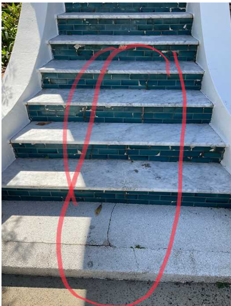
+ Example of cracking to porch stairs. Engage engineer for advice to control and prevent further cracking.
