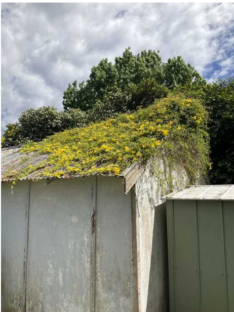
+ Vegetation to roof on garage. Engage roofer to clean and remove to prevent further deterioration of garage roof.
